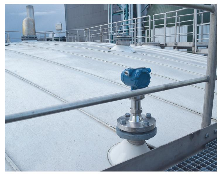
the signals are very low, which makes them unreliable. However, Södra solved this by installing Rosemount 5408 Non-Contacting Radar Level Transmitters with parabolic antennas.
