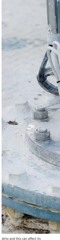
dirty and this can affect its performance. The latest radar transmitters can detect a dirty antenna using signal quality metric diagnostics, enabling preventative maintenance to be scheduled.
