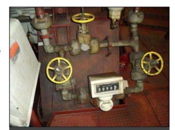
During a class energy-profiling exercise, the old fuel flow meters (above) for the four main engines aboard Military Sealift Command dry cargo/ammunition ship USNS Robert E. Peary were replaced by new meters with sensors that measure fuel usage per minute (below). Readouts quickly gauge fuel consumption.
