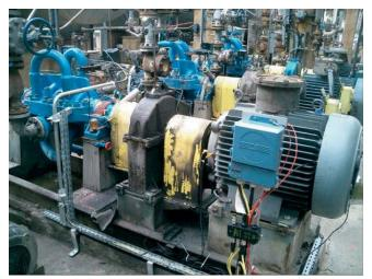
High vibration due to a bearing problem can typically be isolated to a specific bearing location, while vibration due to cavitation can be detected at every pump measurement location.
