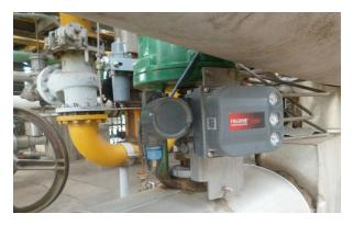
On the back side of the valve is a FIELDVUE DVC6200 digital valve controller with online monitoring and Advanced Diagnostic capabilities.
