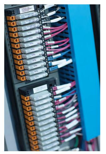
TPC Group, for example, is in the midst of a staged modernization of the control systems at one its Gulf Coast petrochemical facilities. They're transitioning a few process units at a time over to the DeltaV system, and ultimately will Electronically Marshal all of their I/O. "And we're not taking any of our processes down," notes Bob Crawford, staff engineer in the company's process automation group. "It'll be hot cut-over on more than 5,000 I/O when all's said and done."
