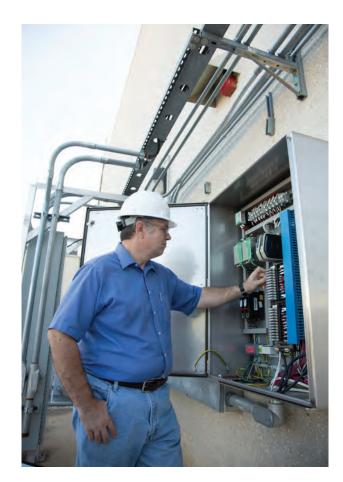
We just lifted the wires off the old I/O card, landed them on the new terminals, and—boom—it was talking.
