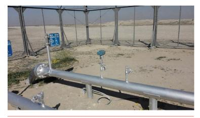
**Figure 2.** A wireless gateway and an RTU panel collect data from pressure, temperature,  $H_2$ S and  $CH_4$  transmitters. The RTU also interfaces with the pump controller and the downhole gauge.
