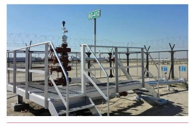
**Figure 1.** This lift station is similar to many others used by KOC. A wireless transmitter measures wellhead pressure, and a second wireless transmitter measures wellhead temperature. Readings from these and other devices are transmitted to and shown in the main control room.
