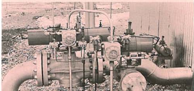
Three Robotarm Actuators, Models 732, 701 and 301, controlling discharge, bypass and vent valves on a gas turbine-driven compressor.
