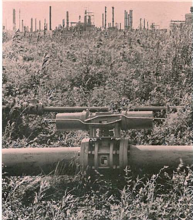
Three Robotarm Actuators, Models 732, 701 and 301, controlling discharge, bypass and vent valves on a gas turbine-driven compressor.
