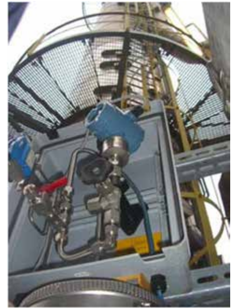
The Rosemount 3051ERS System improves both accuracy and reliability of the level measurement on the distillation column, while cutting response time by 90%.
