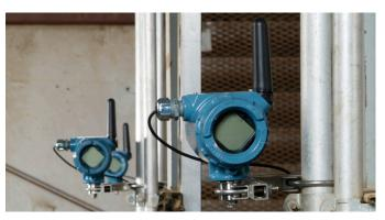
• The AMS 9420 delivers critical vibration information directly to the control room to help operators identify potential production risks.
