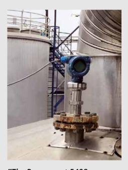
"The Rosemount 5408 was able to handle turbulence, foam, and agitators and provide a reliable, stable level measurement."
