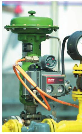
Robust Foundation Fieldbus cabling networks the digital Fisher control valves that feature 'Control in the Field' capabilities with integral PID control
