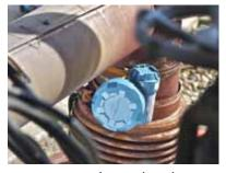
Acoustic noise detected on the safety relief valve of an economizer alerted operators to a potential problem that risked a plant trip.
