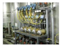
ELITE CMFS015 meters for charging polymer to aging tanks. These fractional sized meters provided best performance balancing accuracy and pressure drop.
