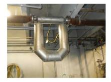
ELITE CMF300 used to measure incoming mud stream. Flow, density and temperature measurements are used to calculate net solids.
