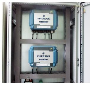
The old communication devices in the control room cabinets were replaced with the Rosemount 2460 System Hub which supports the previous field device communication protocol. Simply plug-and-play using the same cabling.
