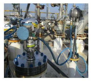
The existing radar level gauge is replaced with a Rosemount™5900S with LPG/LNG antenna and temperature measurement. A second radar level gauge was added to achieve measurement redundancy and improved safety.
