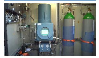
The HyDeploy project uses Rosemount 700XA Gas Chromatograph to provide an independent validation of the full hydrogen and natural gas blend rate.
