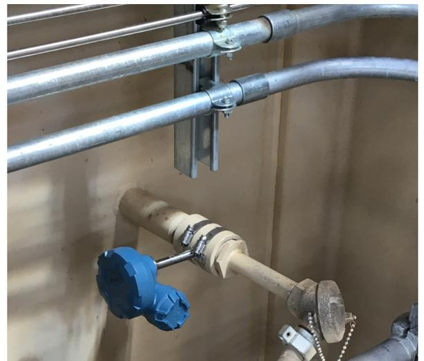
*Rosemount™ 708 Wireless Acoustic Transmitter Provides Non-Intrusive, Real-Time Tube Leak Detection*
