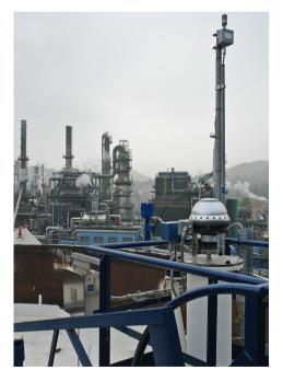
TankRadar Rex installed with a Smart Wireless THUM Adapter.
