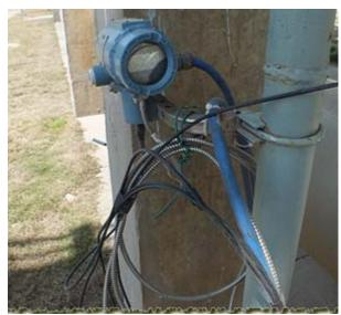
Installed Rosemount 8800 Vortex Flowmeter.
