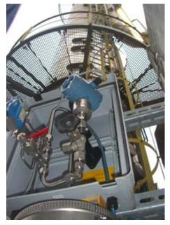
The Rosemount 3051ERS System improves both accuracy and reliability of the level measurement on the distillation column, while cutting response time by 90 percent.
