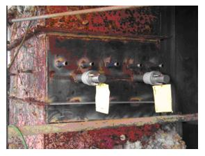
Primary elements and the traverse test points in the duct
