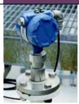
Rosemount 3300 Guided Wave Radar Installed
