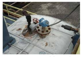
Figure 2: Rosemount 5302 Guided Wave Radar reliably measures emulsion layer on desalter vessel.
