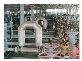
A Micro Motion meter measures the flow of ethylene gas.
