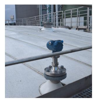
Rosemount 5408 with process seal mounted on a mixing tank
