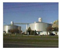
**Image 2.** Sugar silos at ACS in EGF have a rotating bridge that made wired instrumentation impossible to implement.
