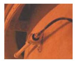
**Image 6.** A remote antenna on the center rotatingshaft inside the sugar silo allows the wireless instruments to communicate with the Wireless Gateway located outside each silo.
