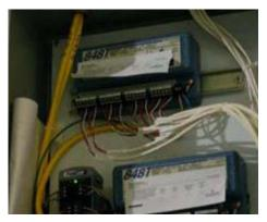
Image 4. One Rosemount 848T Wireless Temperature Transmitter can handle up to 4 inputs including 4-20mA, mV, Thermocouple, RTD, or ohm. The field hardened enclosures and intrinsically safe Power Module makes it ideal for this hazardous environment.
