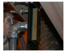
**Image 1.** Rub blocks provide an indication when the conveyor is even slightly out of alignment. A conveyor out of alignment can be a potential ignition source.
