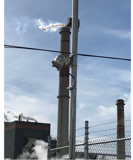
The horn and strobe are mounted on the pole with the Incus.
