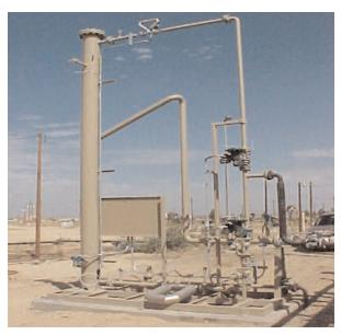
Two Micro Motion Coriolis flowmeters replace costly three-phase test separators, enabling an oil producer to conduct accurate daily well tests.
