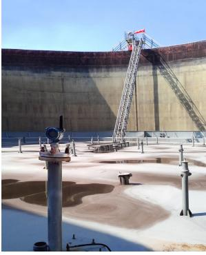
Climbing tanks is no longer required to check the status of the floating roof. Supporting features within the Rosemount TankMaster software enables automatic roof monitoring.
