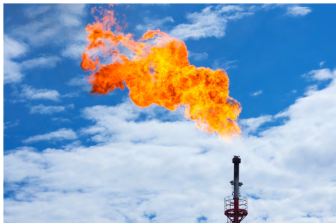
Figure 4.6: A refinery or petrochemical plant flare.
