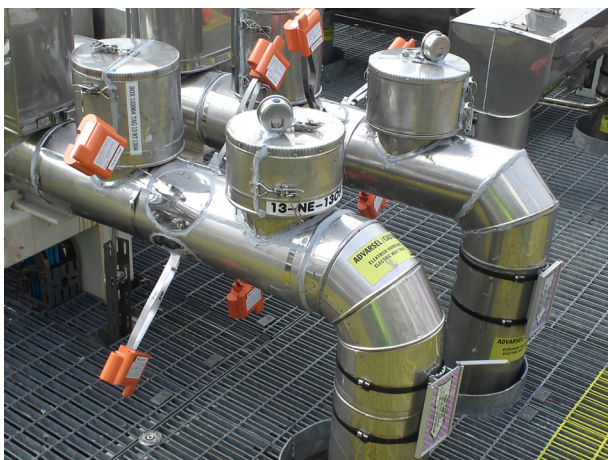
Figure 5. Permasense WT210 ultrasonic sensors can monitor corrosion on a real time basis, allowing refineries to measure the effectiveness of corrosion control methods.
