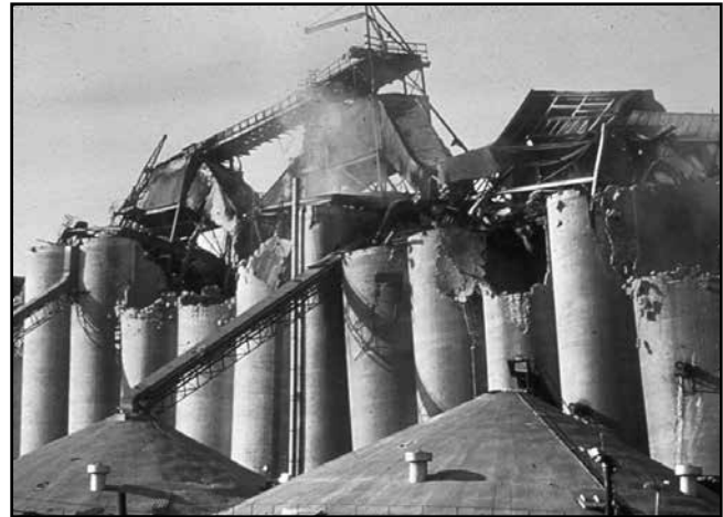
ELIMINATING DISASTERS LIKE THIS REQUIRES CAREFUL CLASSIFICATION OF AREAS AND THE USE OF THE PROPER ELECTRICAL EQUIPMENT.
