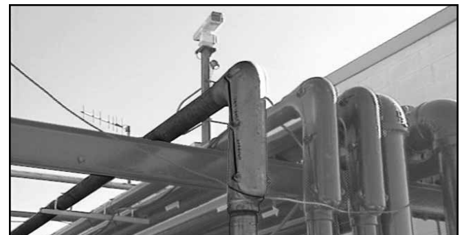
TYPICAL CLASS I, DIVISION 2 RIGID CONDUIT INSTALLATION.
