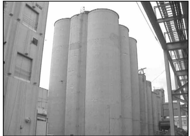
GRAIN ELEVATOR — CLASS II, DIVISIONS 1 AND 2.
