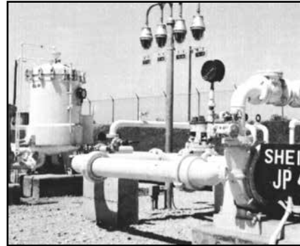
INSTALLATION OF LUMINAIRES IN JET FUEL AREA.
