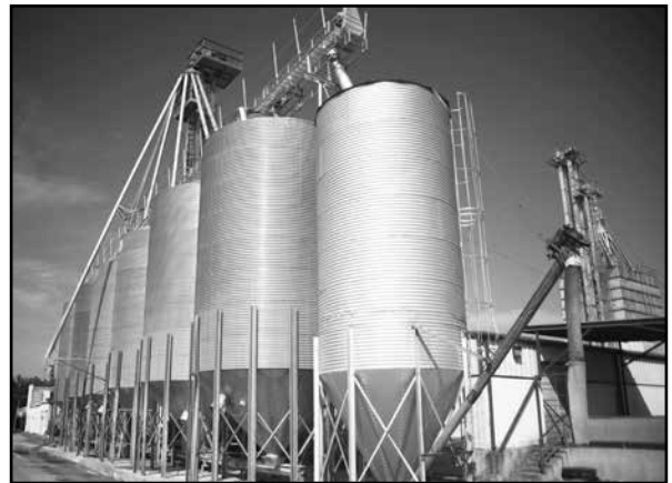
CLASS II, DIVISION 1 AND 2, GROUP G GRAIN ELEVATOR.
