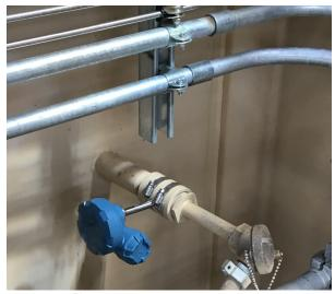
Rosemount<sup>™</sup> 708 Wireless Acoustic Transmitter Provides Non-Intrusive, Real-Time Tube Leak Detection
