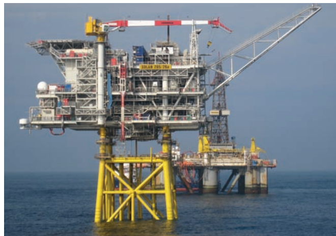
The Solan platform will be unmanned and controlled via satellite link from an onshore control room, with monthly visits for inspection and maintenance. (Photo courtesy Premier Oil)
