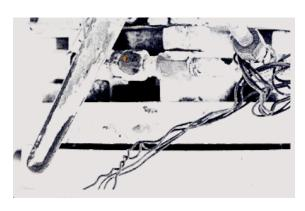
WIRES LIKE THIS INDICATE A LACK OF VALVE MAINTENANCE. THEY ARE USED TO HOLD THE OPERATING LEVER OPEN-A VERY BAD PRACTICE.
