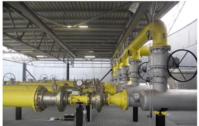
Figure 3: Axial Flow Pressure Regulators equipped with RAF system
