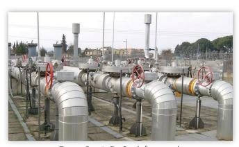
Toscana Energia City Gate before upgrade 6" Top Entry Regulators without Integrated Silencers With wall panels & pipe insulation
