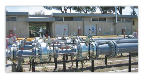
6" FL Wide-Open Monitors and 6" FL/SRS Regulators installed in Toscana Energia City Gate, Ugnano Florence, Italy
