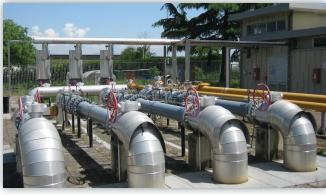
Toscana Energia City Gate after upgrade 6" FL Axial Flow Regulators with Integrated SRS Silencers Without wall panels and pipe insulation
