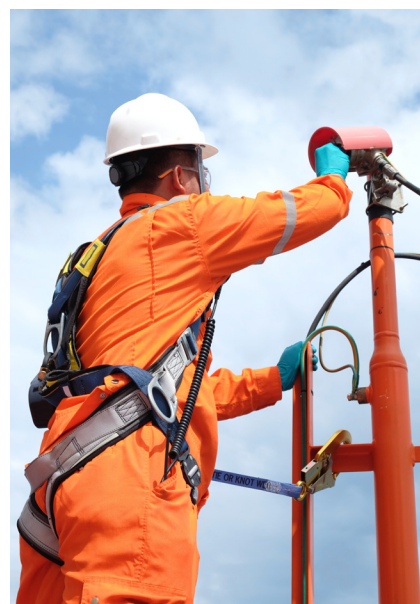
Figure 3: Flame detectors should be placed selectively around hazardous areas where there is potential for flammable products to escape.
