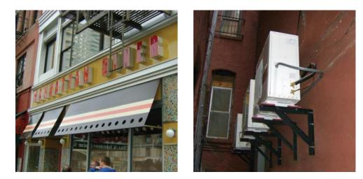
Manhattan Diner, located in NYC at 94th & Broadway, could not install conventional condensing units on the roof of its six-story building due to space constraints. A seven-foot wide alley was the only other location option. The X-Line condensing unit's **slim profile allowed the units to be installed safely on the building** wall using heavy-duty brackets – high enough not to interfere with the ground areas between New York City's alleyways.
