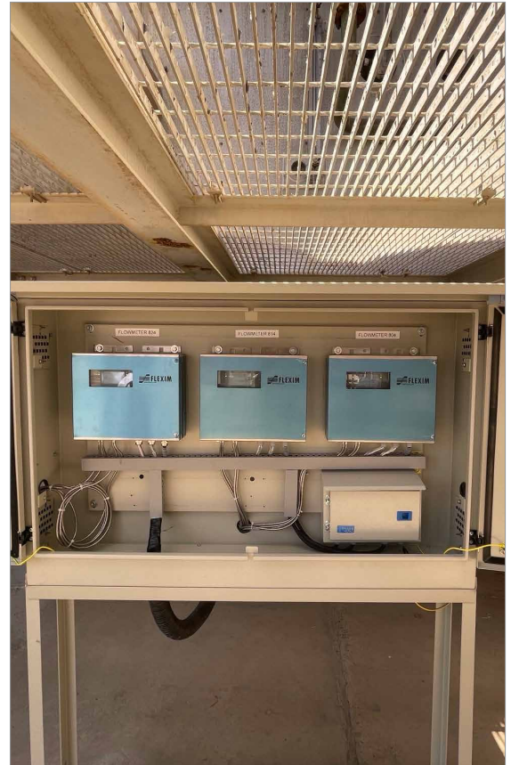
Dual-channel versions of the FLUXUS® F721 stationary ultrasonic systems are used as transmitters.
