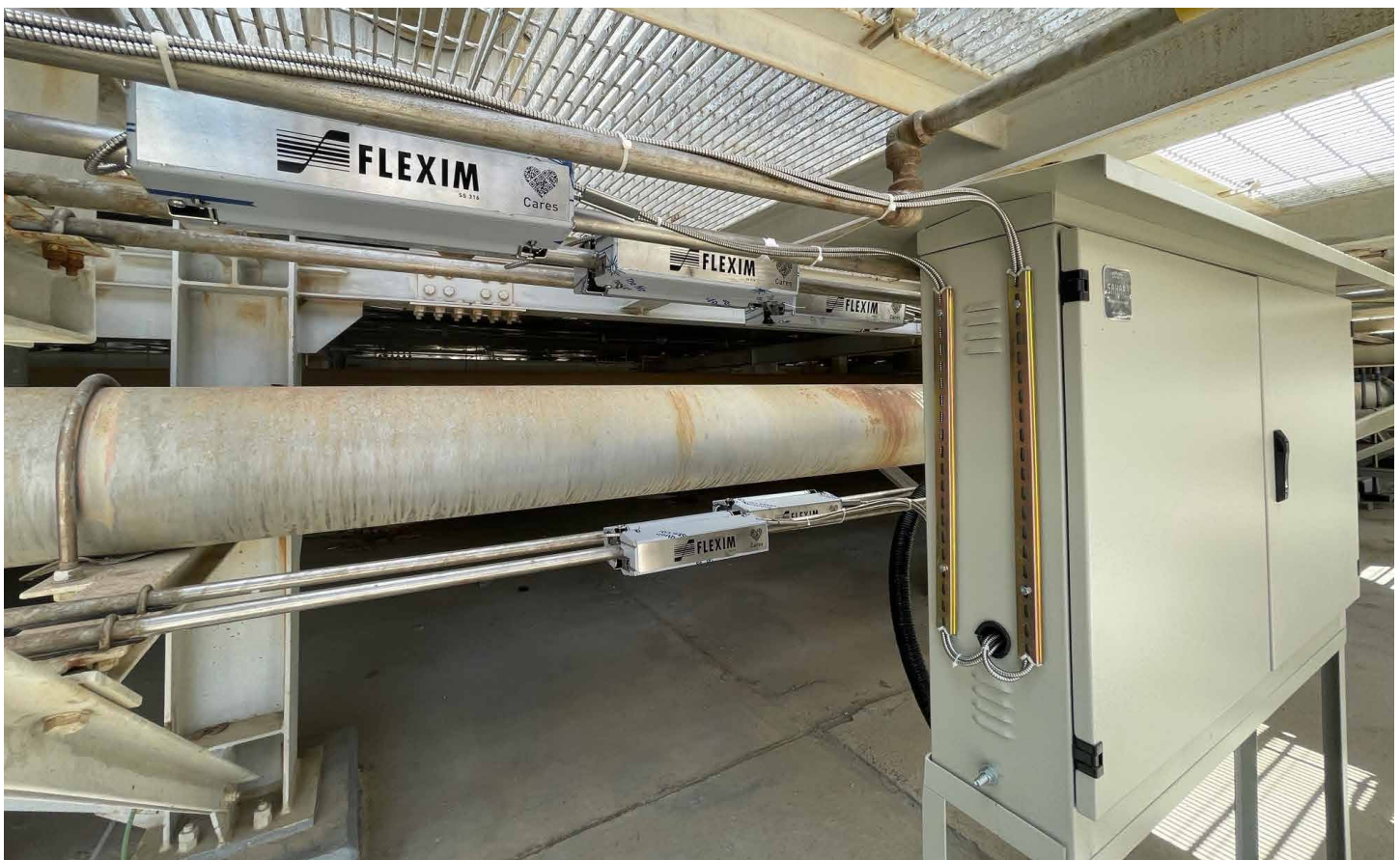
Dual-channel versions of the FLUXUS® F721 stationary ultrasonic systems are used as transmitters.
