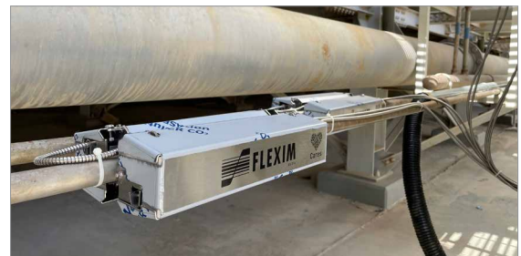
The Variofix C transducer mounting devices provide the transducers mounted in them with a permanently firm hold and protection.
