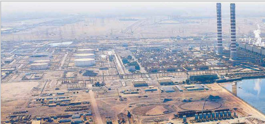
El Sabiya Power and Water Distillation Station is the largest power and water provider in Kuwait. © MEW
