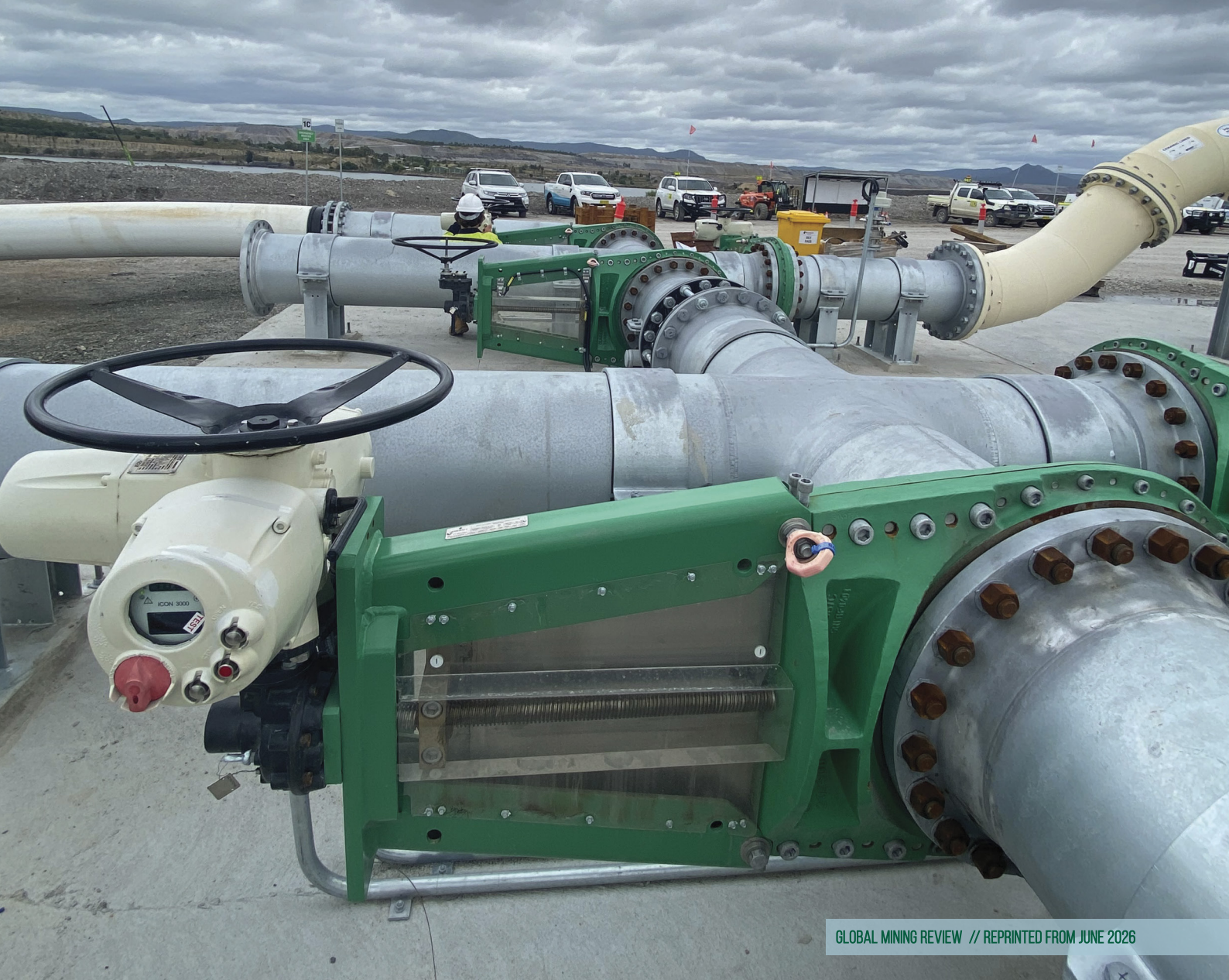
Figure 1. Detail of Clarkson knife gate valve with Bettis XTE actuator.
