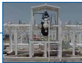
Skid Fabrication and MPFS Integration
