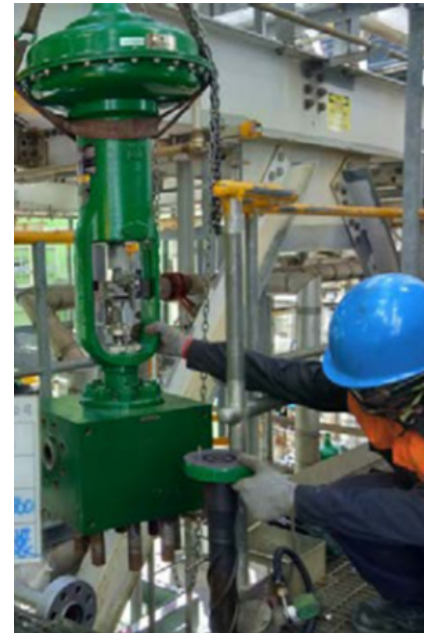
Fisher DFA desuperheater with Micro-Flat trim
