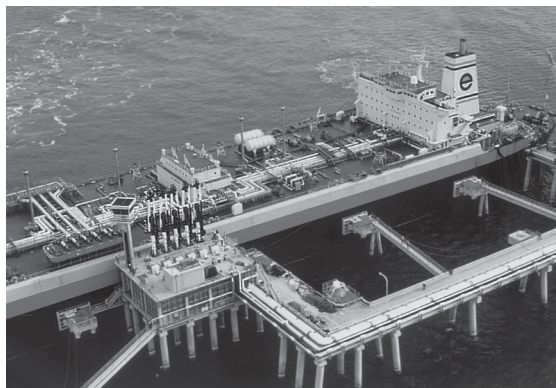
Figure 1. Marine Vapor Control System Application
