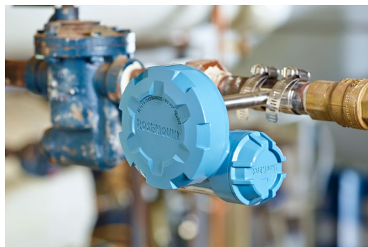
FIGURE 18 Mounting an acoustic transmitter on a pipe adjacent to a steam trap can determine if it is functioning properly, and the transmitter can report its results to the reliability team.
