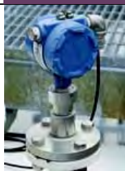
Rosemount 3300 Guided Wave Radar Installed
