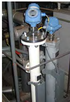
Figure 2. A second Rosemount 5301 replaces the electronic displacer.
