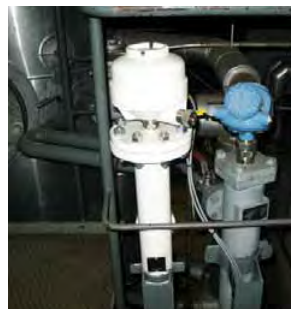
Figure 1. Rosemount 5301 replaces a displacer on chamber for condenser level control.
