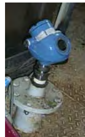
Figure 2. Installation of Rosemount 5303 Guided Wave Radar.
