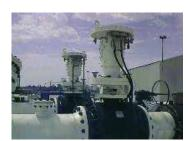
Rotary vane double-acting actuator
